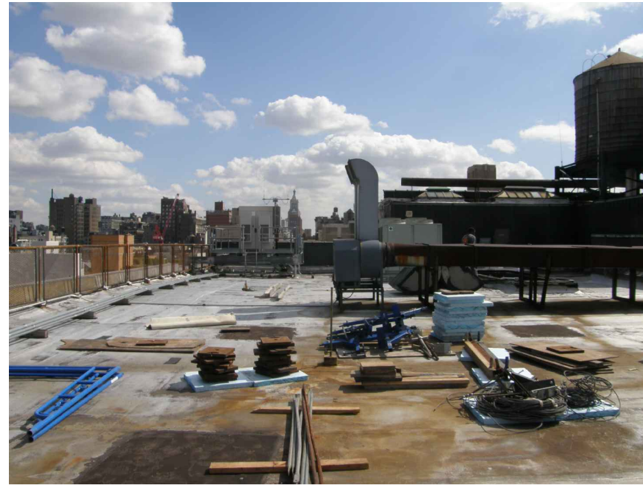
2 EXISTING ROOFTOP EQUIP. EXISTING
