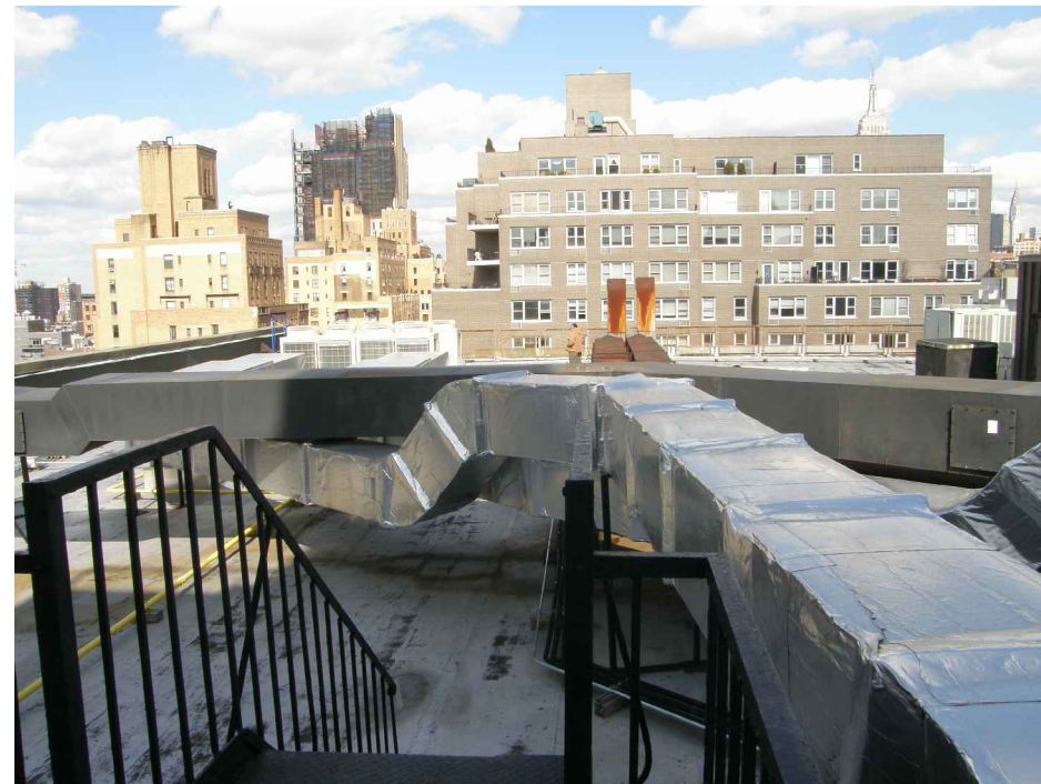
4 EXISTING ROOFTOP EQUIP. EXISTING
