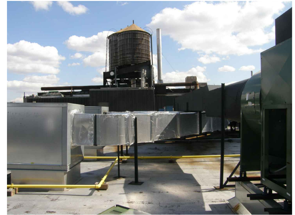
3 EXISTING ROOFTOP EQUIP. EXISTING
