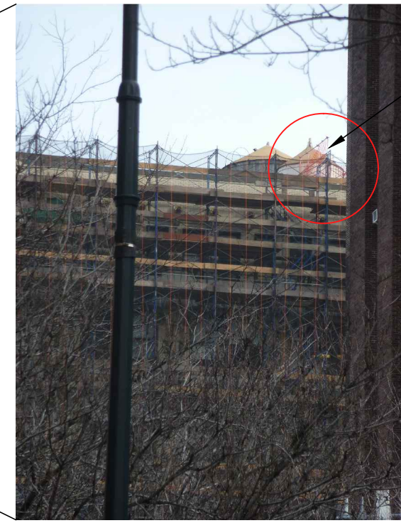
3 DETAIL PHOTO MOCK-UP
