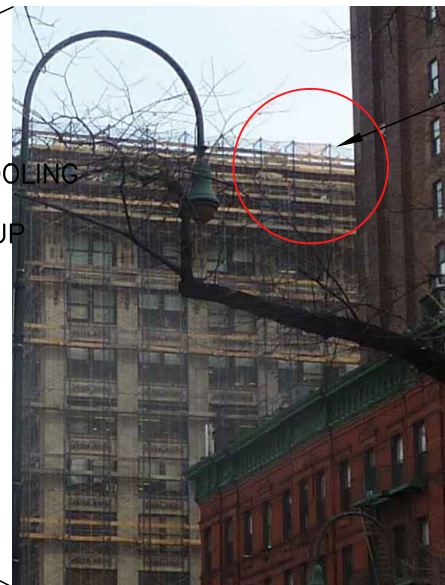
5 DETAIL PHOTO MOCK-UP
